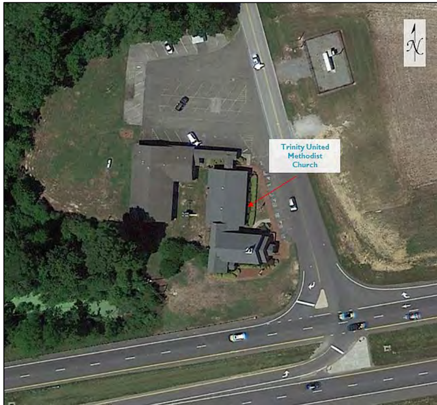
Figure 93: Site plan of Trinity United Methodist Church with US 70 at bottom (base image courtesy of Google Earth).
