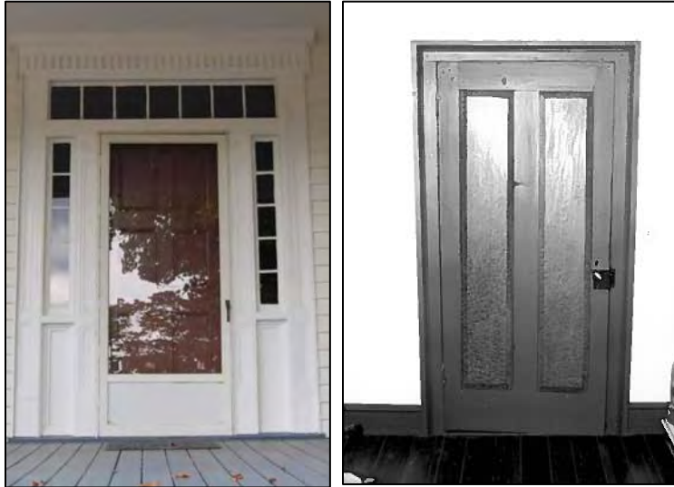
Figure 21: Wiley Joel Rouse House: Federal six-panel door within Greek Revival trabeated surround at front entry, at left, 2017; and Greek Revival two-panel door, at right (photographer: Robbie Jones, 1994).
