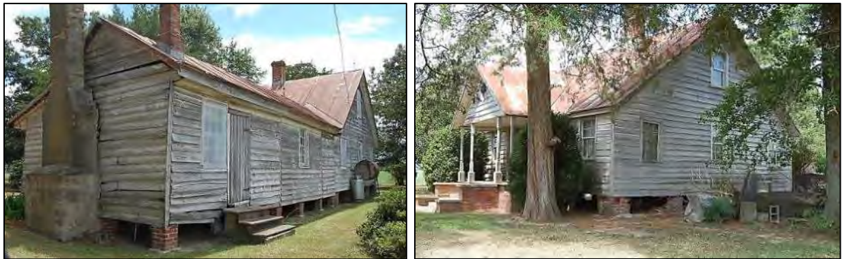
Figure 194: Hines-Warters-Adkinson House: at left, north rear and west side elevations with location of former breezeway to kitchen visible at central window bay; at right, south front and east side elevations, 2017.
