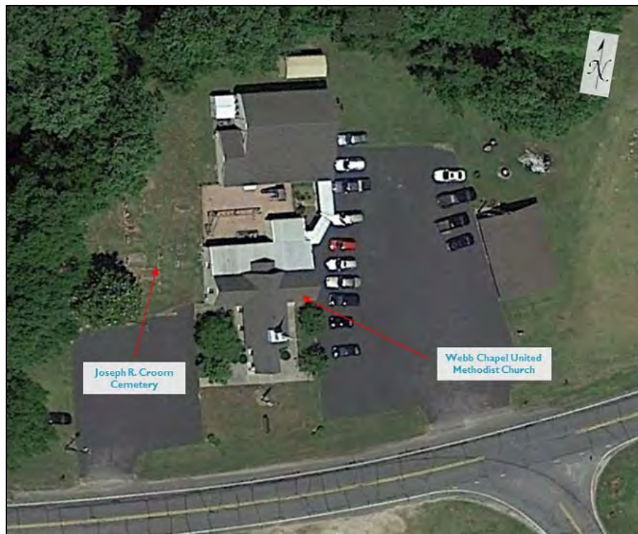
Figure 161: Site plan of Webb Chapel United Methodist Church (base image courtesy of Google Earth).
