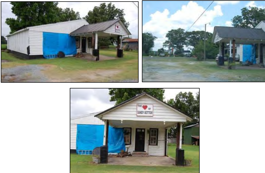
Figure 130: Bessie Croom Stroud Store: top left, west side and north front elevations; top right, north front and east side elevations with former school/Stroud House visible behind canopy and Taylor House in distance; bottom, store front with canopy.
