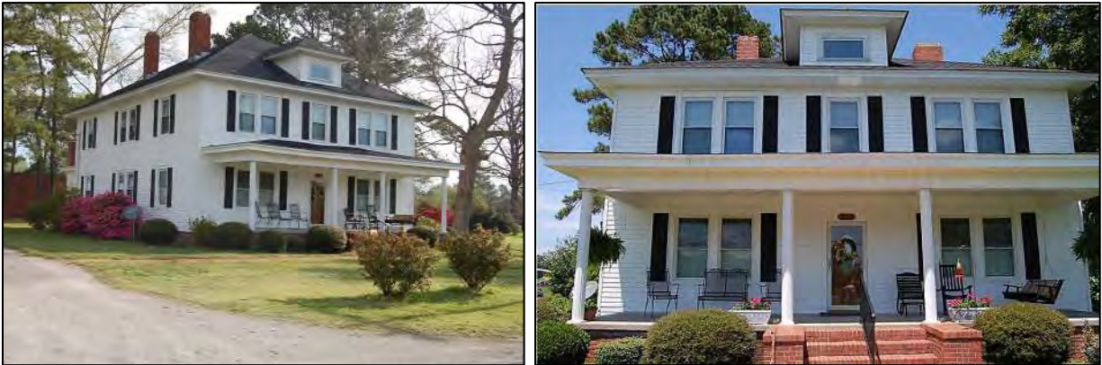
Figure 336: Dover Teacherage: west side and south front elevations, at left; south front elevation, at right
