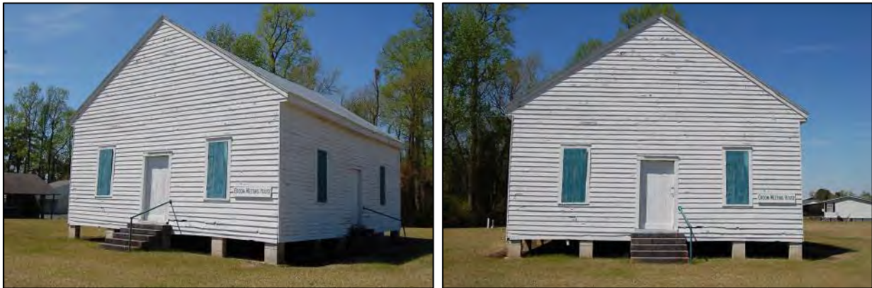
Figure 166: Croom Meeting House: at left, east side and south gabled elevations; at right, south gabled elevation.
