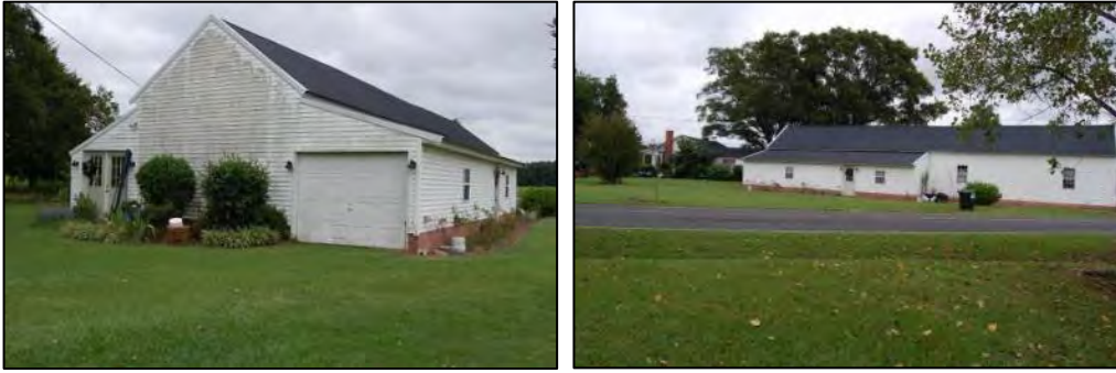
Figure 127: Former Taylor Store: at left, view looking south; at right, view looking northeast with Taylor House in distance.
