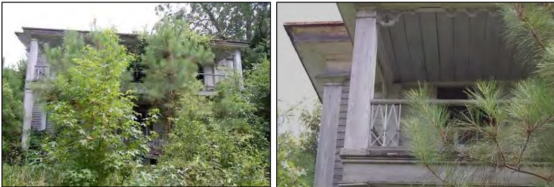
Figure 26: Rouse-Edmondson-Wilson House: front elevation with two-tier porch and porch detail, 2017.
