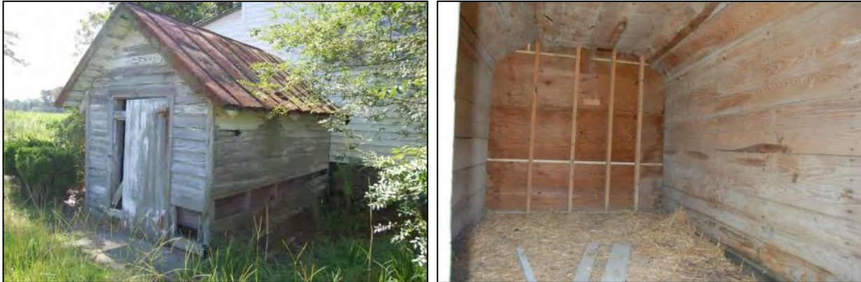
Figure 77: Left, view of northern elevation of shed, looking to south; right, view of interior of shed, looking south.
