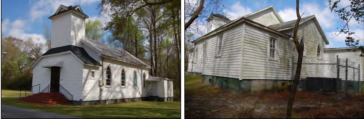
Figure 68: Banks Chapel: at left, south front and east side elevations; at right, east side and north rear elevations with original apse at center.
