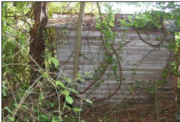
Figure 269: View of shed's southern elevation.
