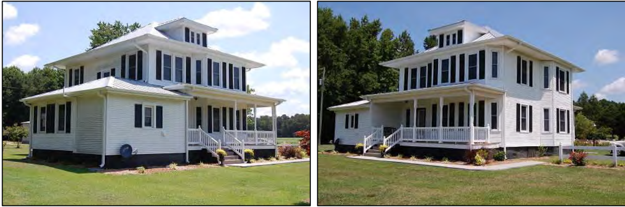
Figure 201: Simpson Waller House: west side and south front elevations, at left, and south front and east side elevations, at right.
