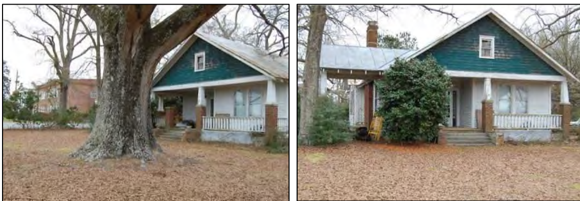
Figure 345: Contentnea School Teacherage: west front elevations of teacherage and Contentnea School, at left, and north side and west elevations of teacherage, at right, 2017
