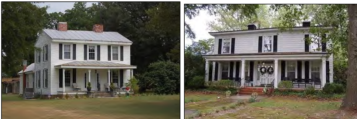
Figure 23: Pridgen-Hardy House, at left, Cunningham-Patrick-Bryan House, at right, front elevations, 2017.
