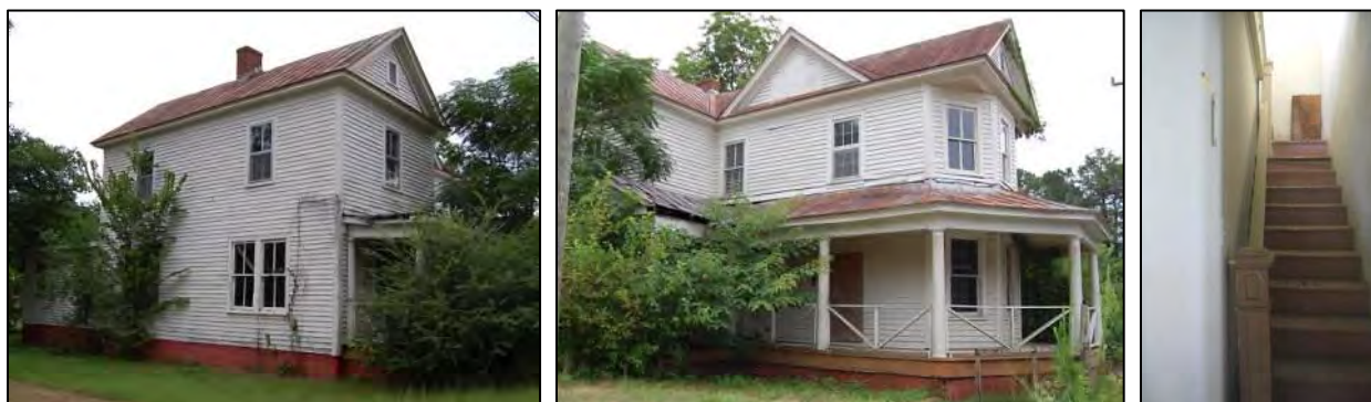
Figure 30: Ezekiel K. Best House: east side elevation, at left, north front and west side elevations, at center, and stair, at right, 2017.
