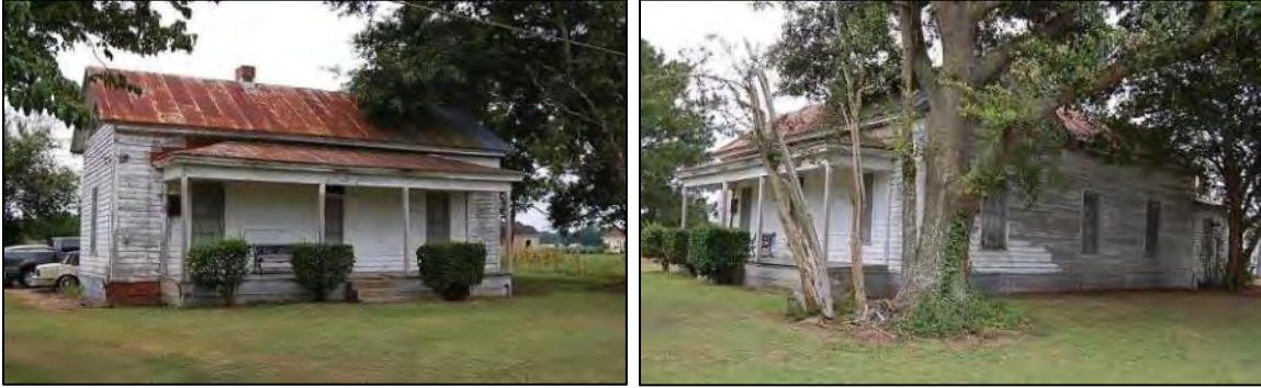
Figure 195: T.J. Herring Tenant House: east side and north front elevations, at left; north front and west side elevations, at right, 2017.
