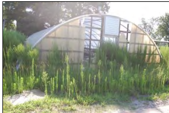
Figure 87: View west at greenhouse.
