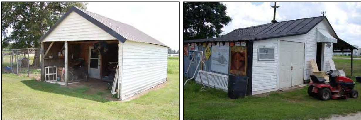
Figure 121: At left, view of garage looking south; at right, view of workshop looking west.
