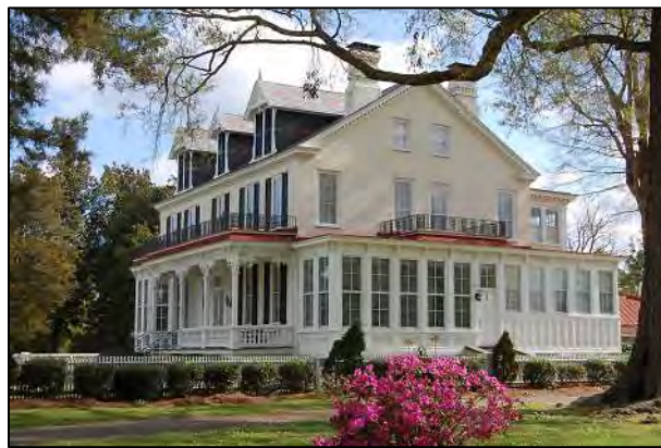
Figure 101: Cedar Dell: west front and south side elevations, 2017.
