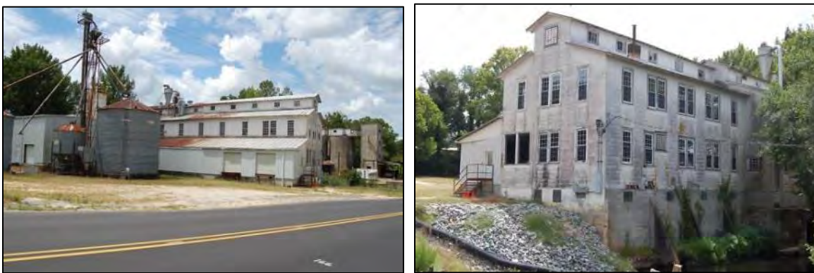
Figure 256: Davis Mill: looking southwest at mill complex, at left, and south and west elevations of mill, at right, 2017.
