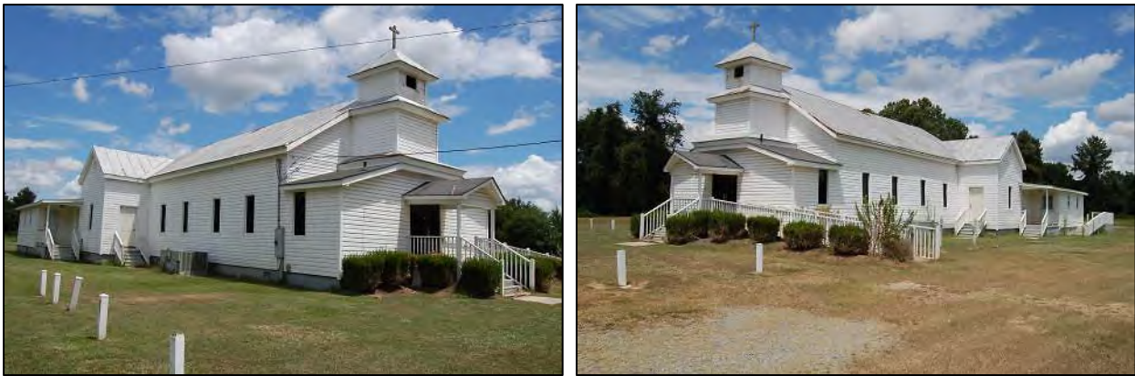
Figure 53: Rockford Chapel: west side and south front elevations, at left, and south front and east side elevations, at right, 2017.
