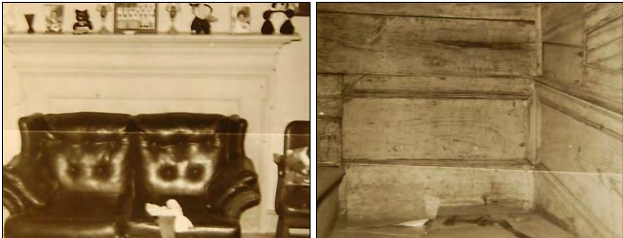
Figure 246: Moseley-Stroud House: late eighteenth/early nineteenth-century mantel in west room, at left, and wainscoting in stair hall, at right, 1993 (Robbie Jones).
