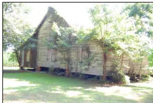
Figure 331: View looking northeast at packhouse.
