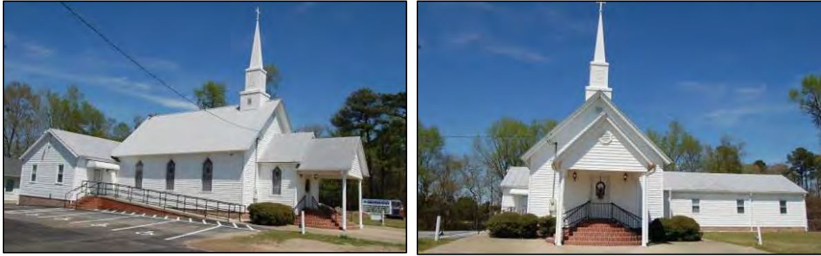
Figure 159: Sandy Bottom Baptist Church: at left, west side and south front elevation; at right, south front elevation.
