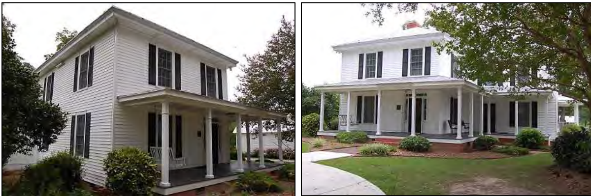
Figure 38: Seth or Willie West House: west side and south front elevations, at left, and south front and east side elevations, at right, 2017.
