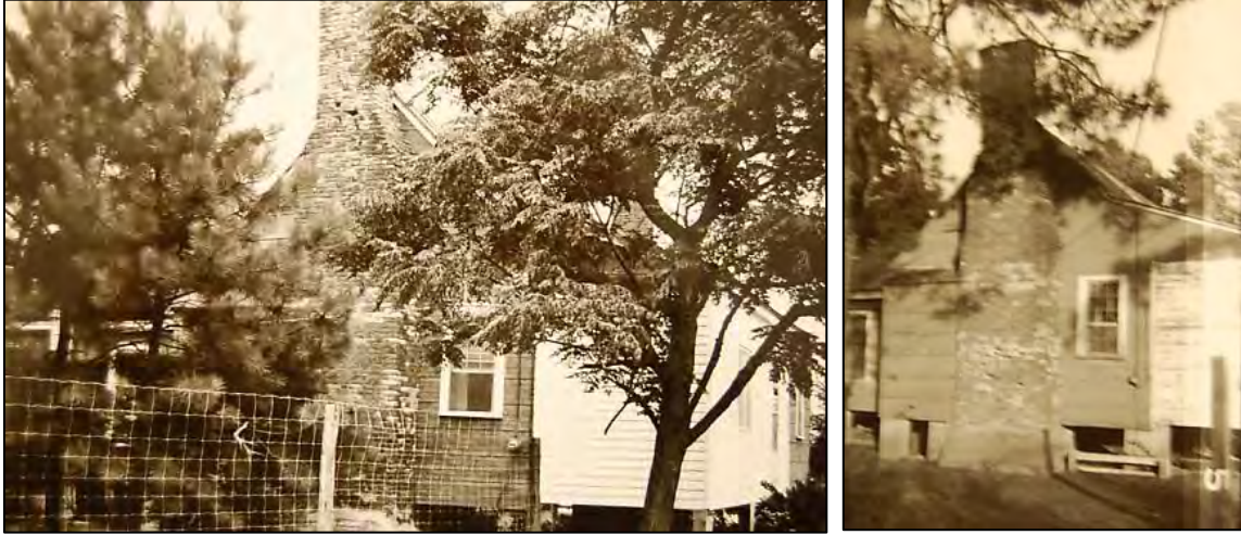
Figure 242: Moseley-Stroud House: west side elevation at left, 1968 (source: North Carolina Division of Cultural Resources), and at right, 1993 (Robbie Jones).
