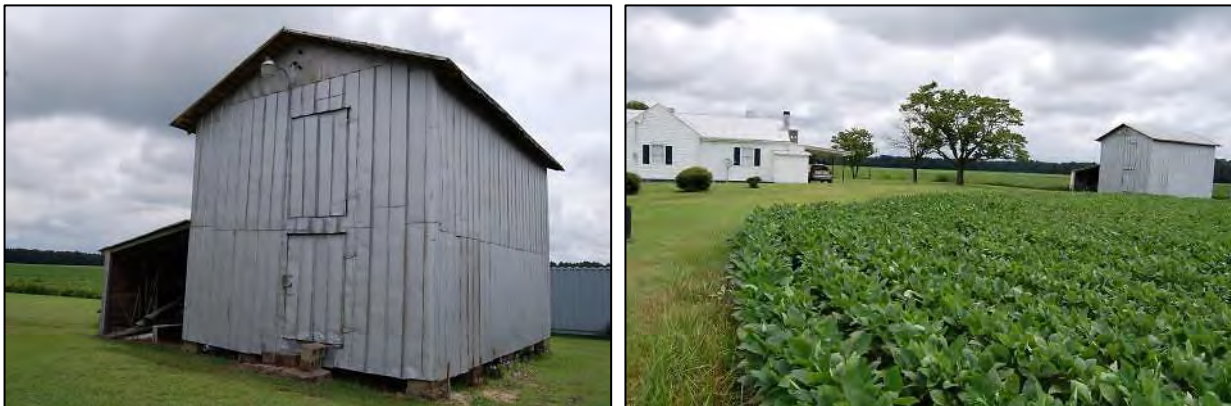
Figure 142: Packhouse: at left, north front and west side elevations; at right, looking east across tobacco fields within the historic district at house to left and packhouse to right.
