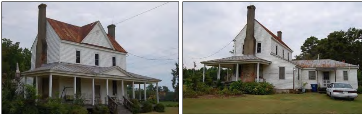
Figure 13: Jericho: west side and south front elevations, at left, and east side and north rear elevations with original shed-roofed ell and turn-of-the-century hip-roofed addition, at right, 2017.
