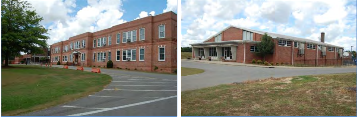
Figure 182: Moss Hill Elementary School: at left, original 1917 block with 2010 addition to its left; at right, 1955 gymnasium, 2017.
