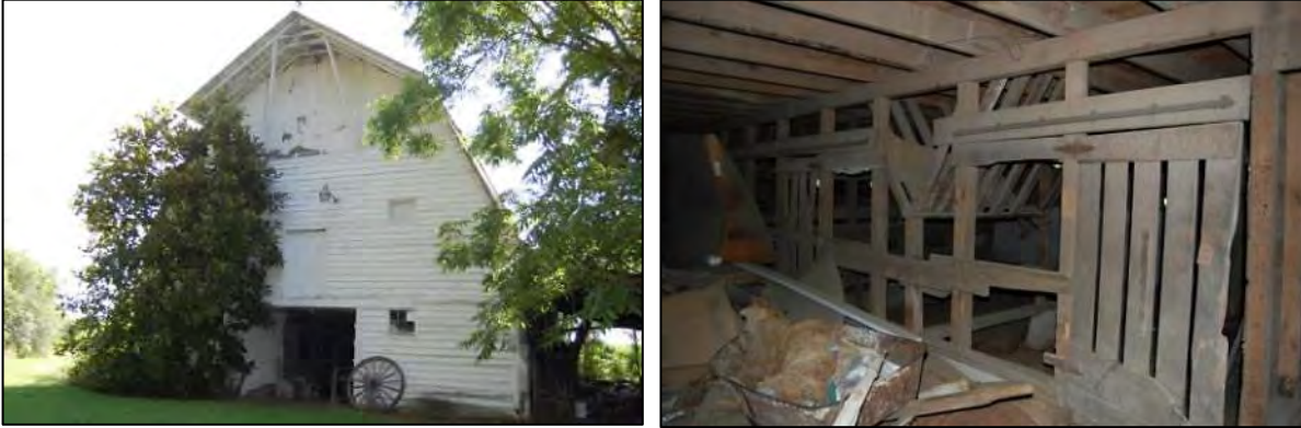
Figure 329: West front elevation of dairy barn and interior stalls retaining feed bins.
