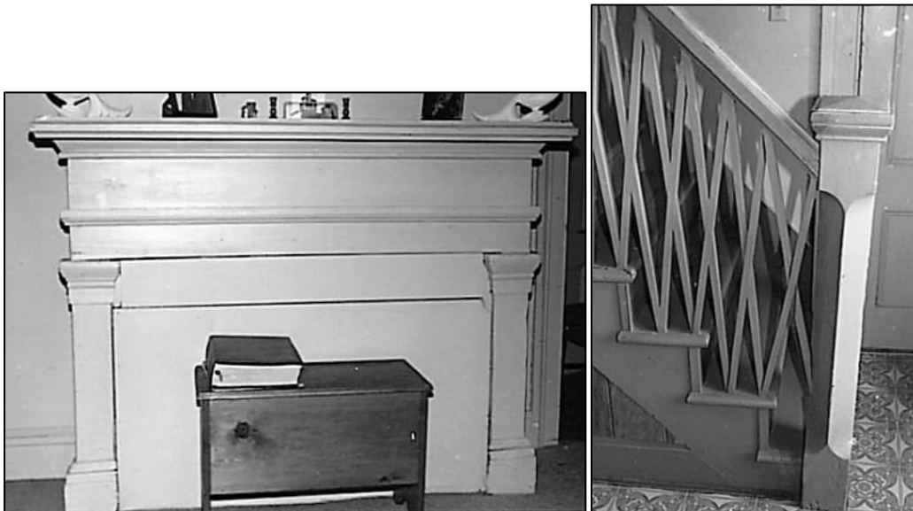
Figure 289: One of four identical post-and-lintel mantels and vigorously modeled stair in 1994 (Robbie Jones)
