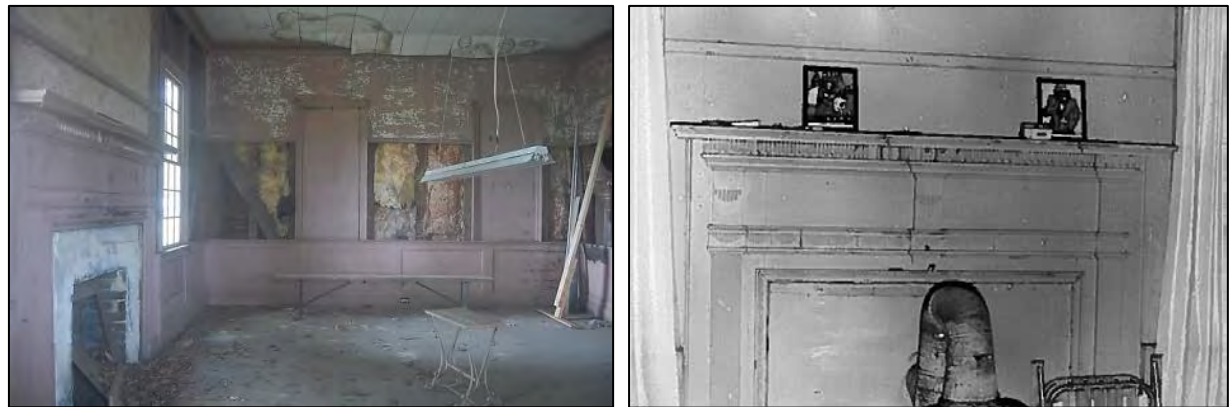
Figure 10: Herring House: west parlor with reeded mantel, flush-paneled wainscoting, and three-part surrounds, 2017; detail of mantel in 1994 (photographer: Robbie Jones).
