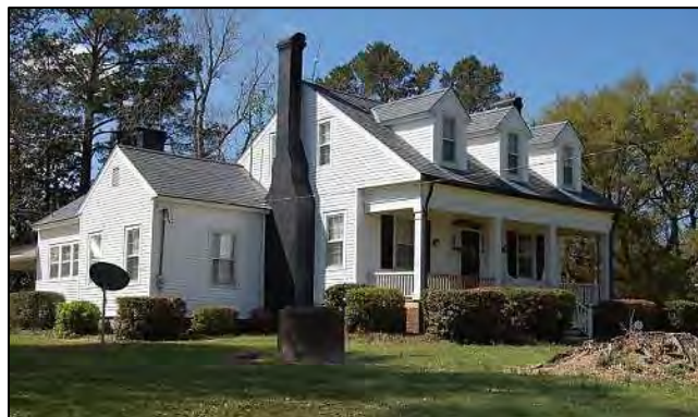
Figure 102: Henry Loftin Herring Farm: east side and north front elevations of house, 2017.
