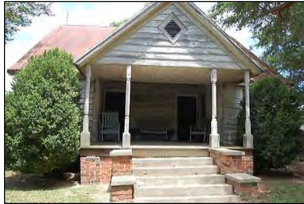
Figure 193: Hines-Warters-Adkinson House: south front elevation with intact recessed entry and ca. 1900 turned columns and porch.
