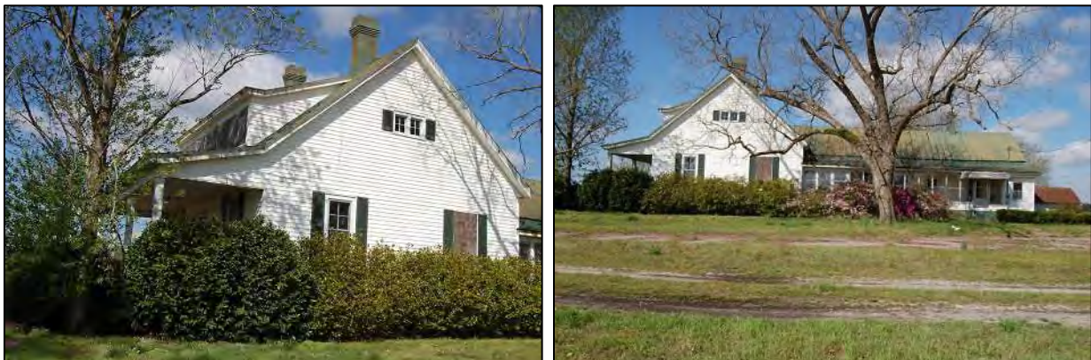
Figure 73: Warters-Parrott-Coleman House: south front and east side elevations, at left; east side elevation, at right.
