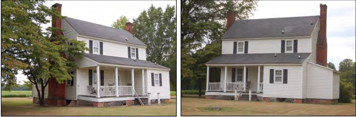
Figure 17: Grady-Harper House: front elevation and double-shouldered chimney, 2017.
