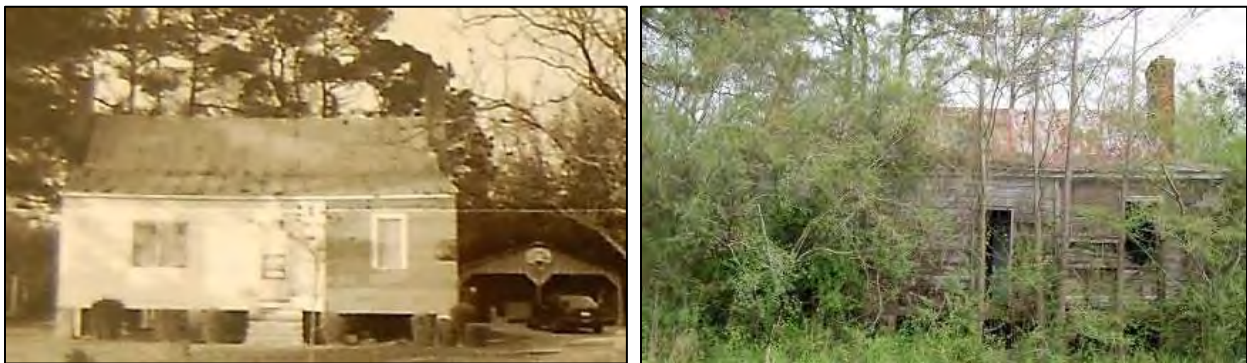
Figure 244: Moseley-Stroud House: south front elevation at left, 1993 (Robbie Jones), and at right, 2017; note that garage is no longer extant.
