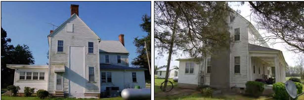
Figure 261: Left, north rear elevation of Cobb-King-Humphrey House; right, west side and south front elevations of house.
