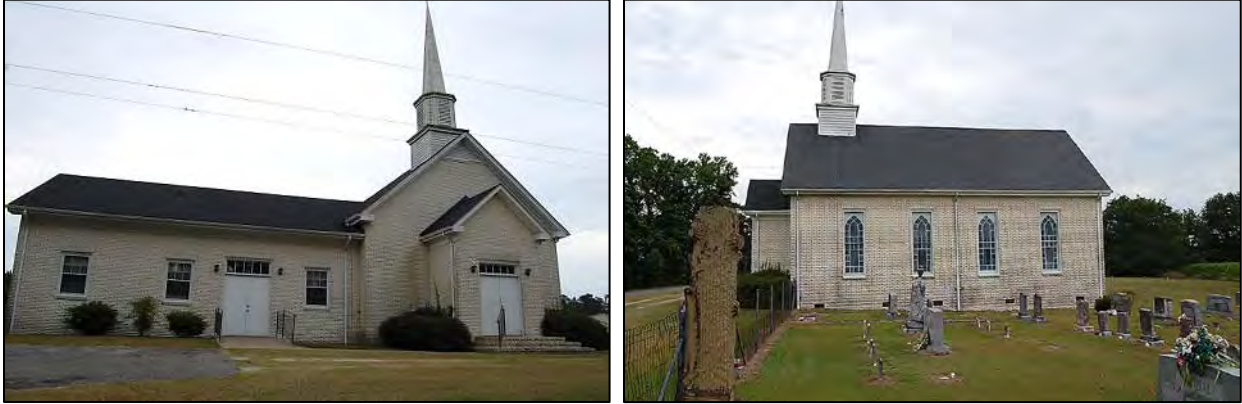
Figure 58: Bethany United Methodist Church: west front elevation with added classroom wing, at left, and south side elevation and cemetery, at right, 2017.
