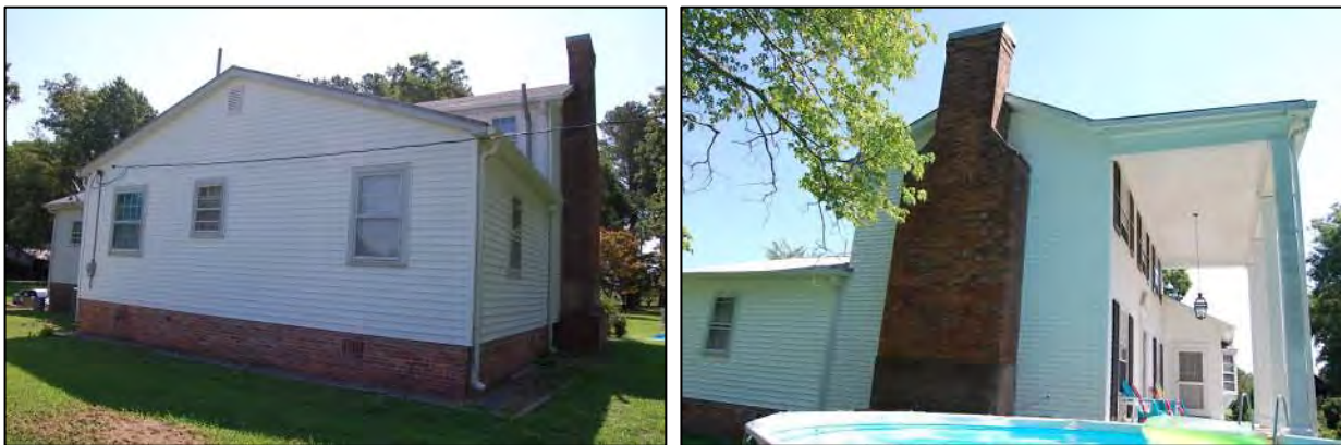
Figure 230: Wilmoth Taylor Sutton House: at left, northwest rear elevation; at right, southwest side elevation with early chimney visible.
