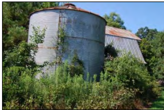
Figure 330: View of grain storage structure, looking southwest.
