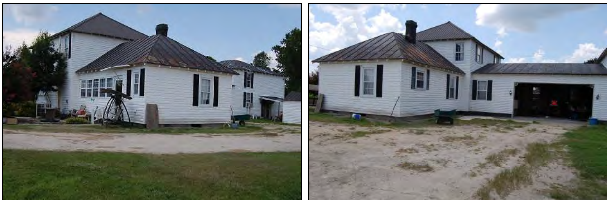
Figure 119: At left, west side and south rear elevations of main block and kitchen ell; at right, south rear elevation of main block and garage hyphen
