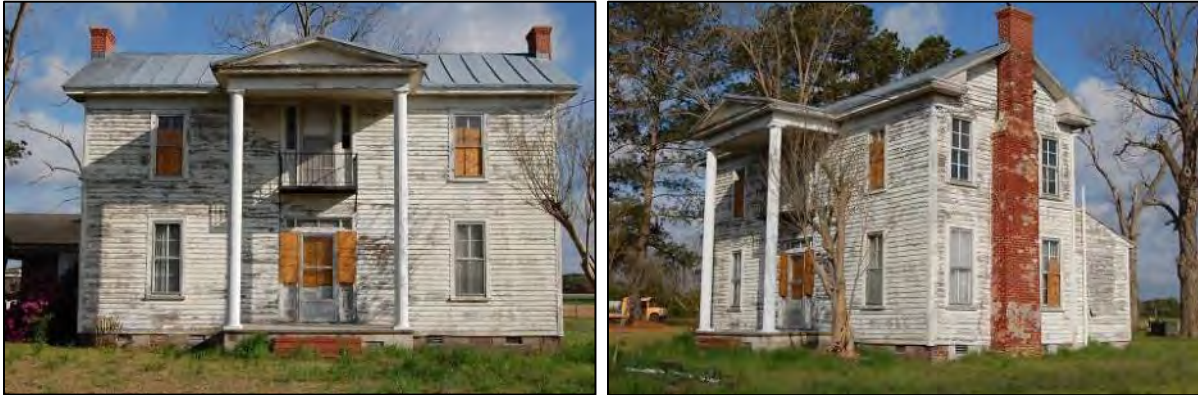
Figure 62: Nathan George Sutton House: at left, south front elevation; at right, south front and east side elevations.
