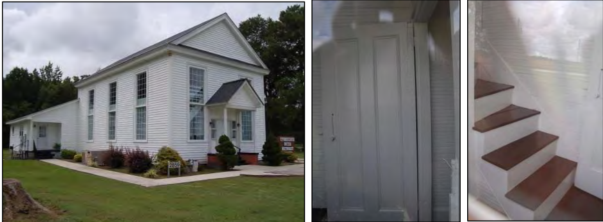
Figure 307: Cypress Creek Methodist Church: northeast side and northwest front elevations, at left, and early door and stair in vestibule, at center and right, 2017.
