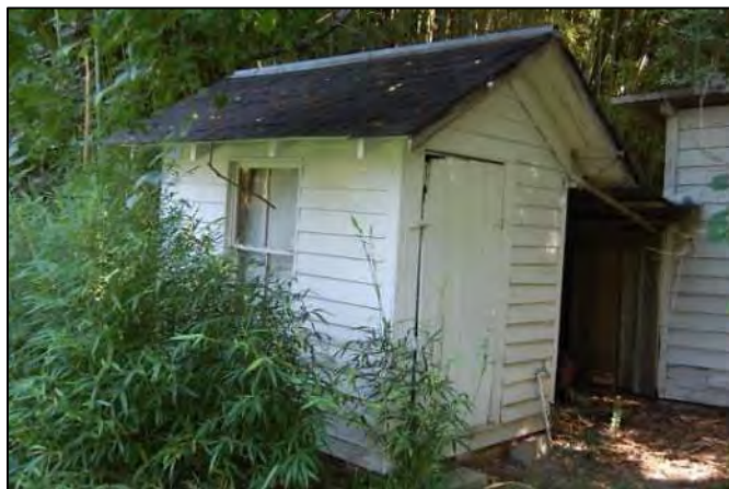
Figure 323: View of southern elevation of brooder house, looking northwest.
