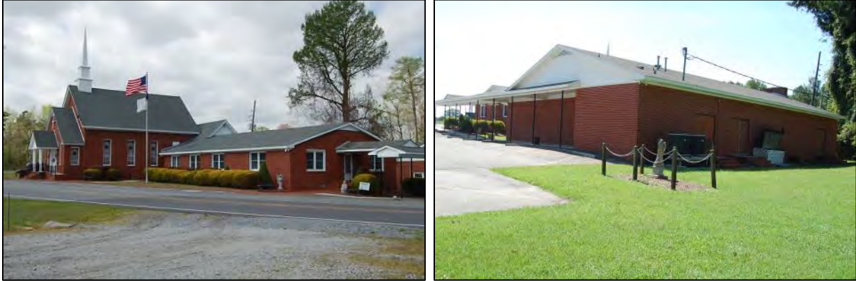
Figure 95: Trinity United Methodist Church: at left, north side elevations of church and addition; at right, east side and north rear elevations of fellowship hall.
