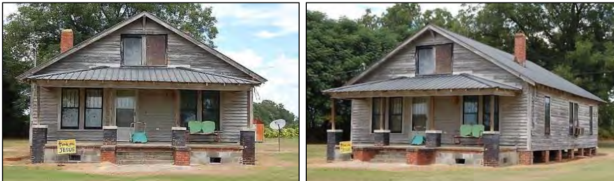
Figure 197: Owen Williams House: south front elevation, at left, and front and east side elevations, at right, 2017.
