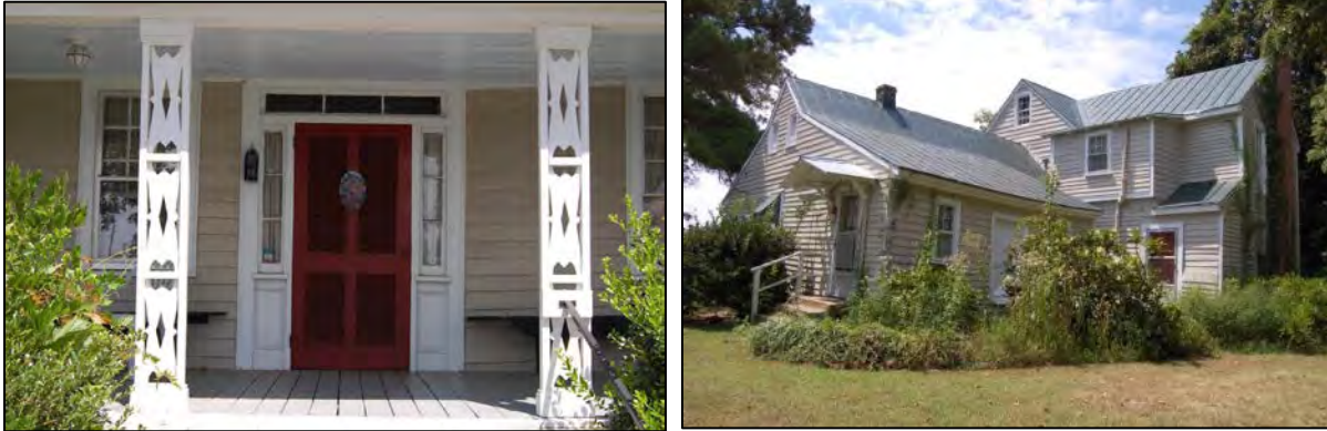
Figure 19: Rountree-Askew-Moseley House: Trabeated entry at principal front block, at left; at right, rear elevation with ca. 1860 block to right, original block to left, and later added/enclosed shed rooms, 2017.
