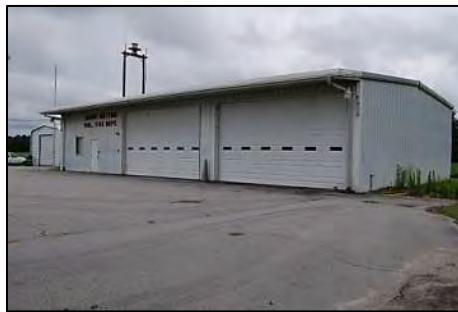
Figure 128: Former Sandy Bottom Firehouse: east elevation.
