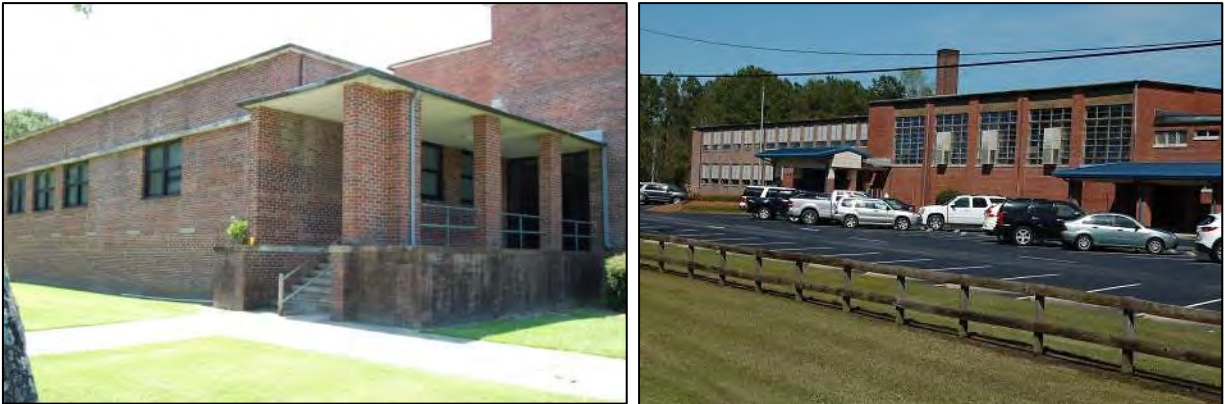
Figure 179: Woodington Middle School: at left, easternmost portion of original block; at right, north front elevations of gymnasium and original block.
