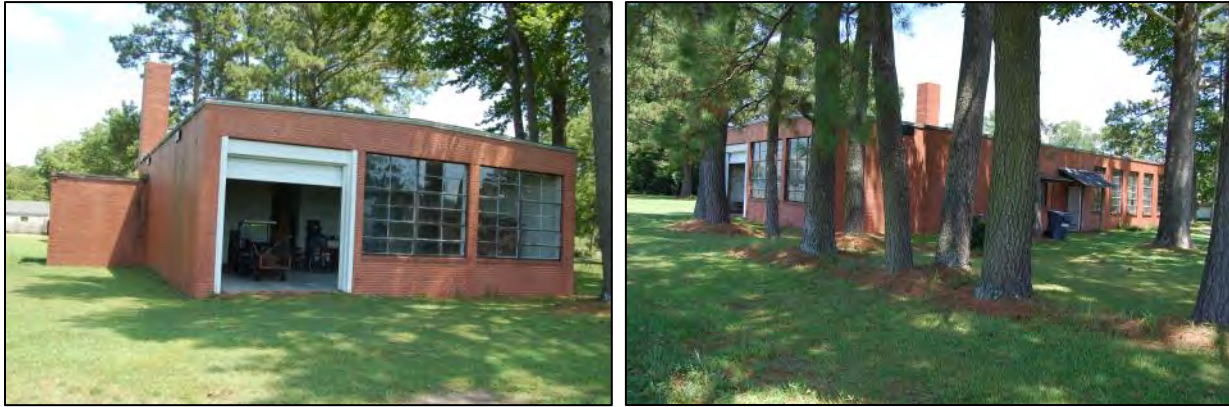
Figure 340: north and east elevations of Vocational Agricultural Building, at left; east and south elevations, at right.
