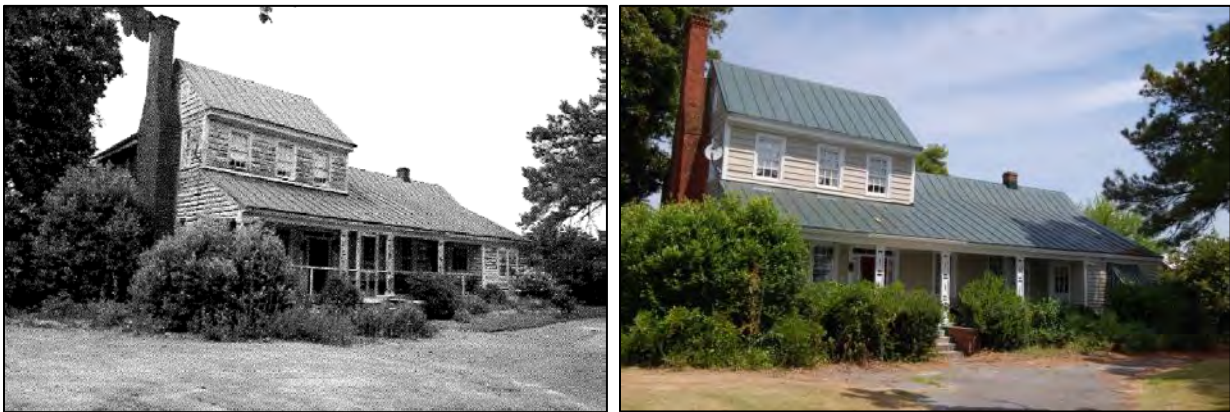
Figure 18: Rountree-Askew-Moseley House: south front and west side elevations in 2010, at left, and 2017, at right.
