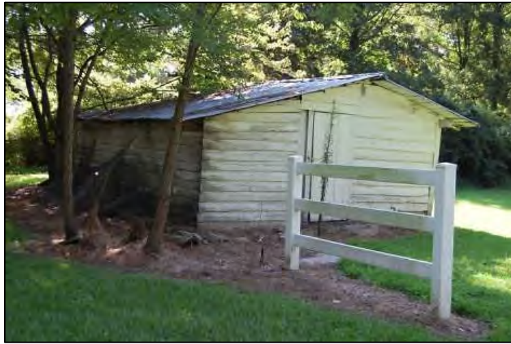
Figure 328: View of southern elevation of Run-In Shed, looking north.
