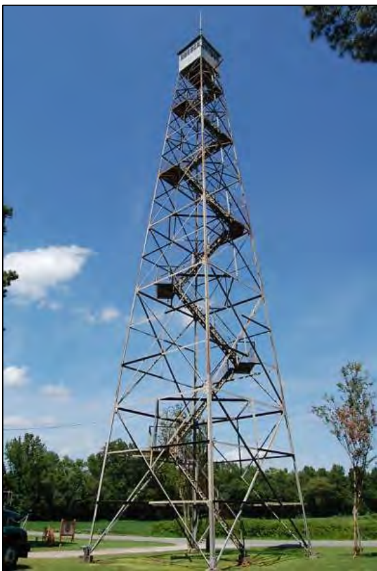
Figure 293: At left, looking northeast at Kelly's Pond Lookout Tower; at right, USDA Forest Service, Region 9, standard plan for 99'9" steel lookout tower with 7' x 7' cab, revised October 8, 1934 (HABS No. M0-1913).
