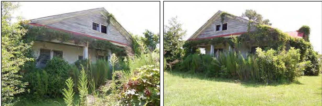
Figure 188: Harper House: west front elevation of Craftsman block, at left, and west front and south side elevations, at right
