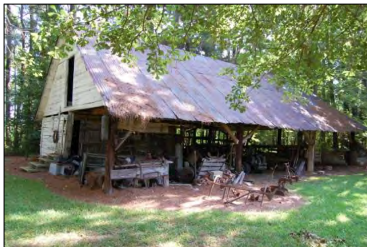
Figure 327: Southern elevation of equipment shed.
