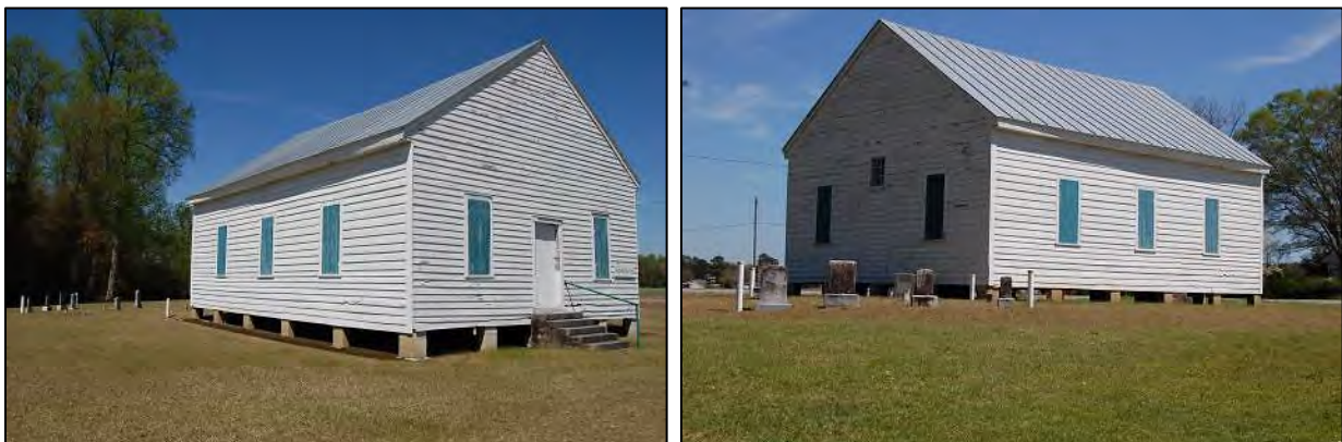
Figure 167: Croom Meeting House: at left, west side and south gabled elevations; at right, north gabled and west side elevations.
