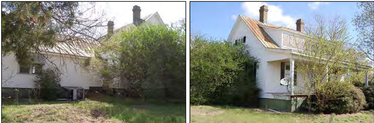
Figure 75: Warters-Parrott-Coleman House: at left, west side elevation with recess that may once have been an open breezeway; at right, west side and south front elevations.
