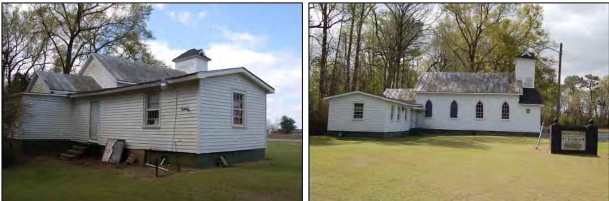
Figure 69: Banks Chapel: at left, north rear and west side elevations; at right, west side elevation.
