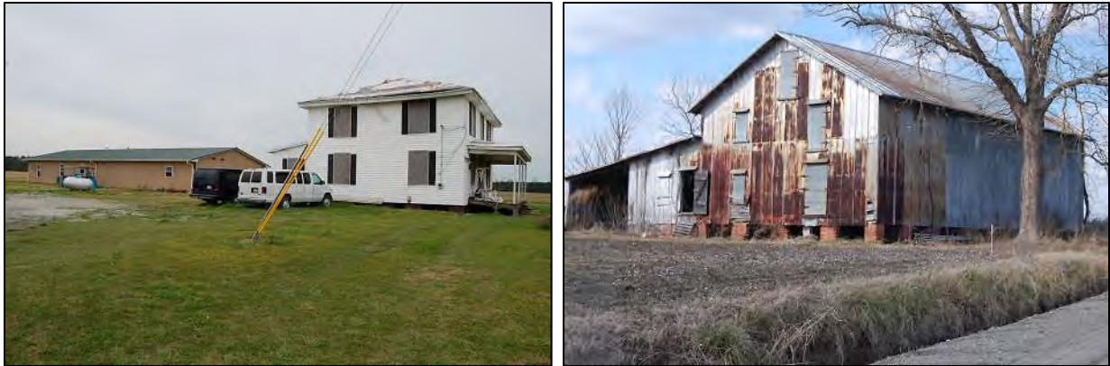
Figure 282: Robert Bond Vause House: at left, view looking southeast of house and modern farm worker housing; at right, 2010 image of large packhouse that no longer stands.
