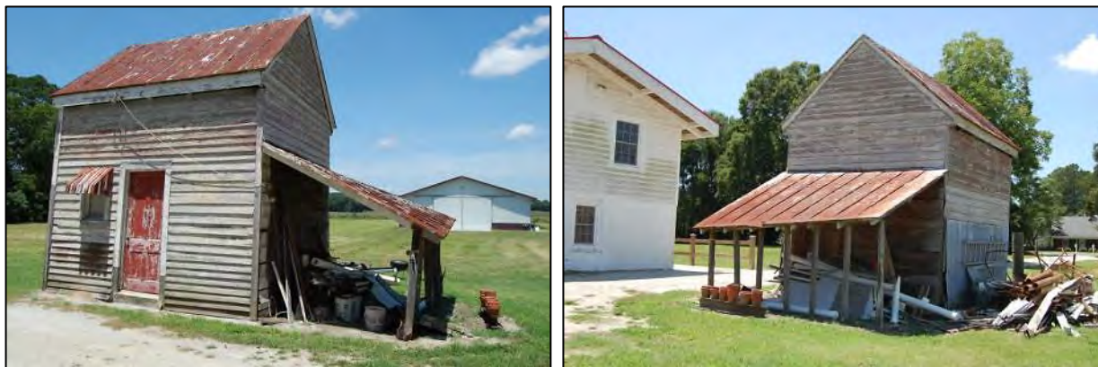
Figure 212: At left, view of south front elevation of smokehouse with modern barn in distance; at right, view of east side elevation of smokehouse with house ell at left.
