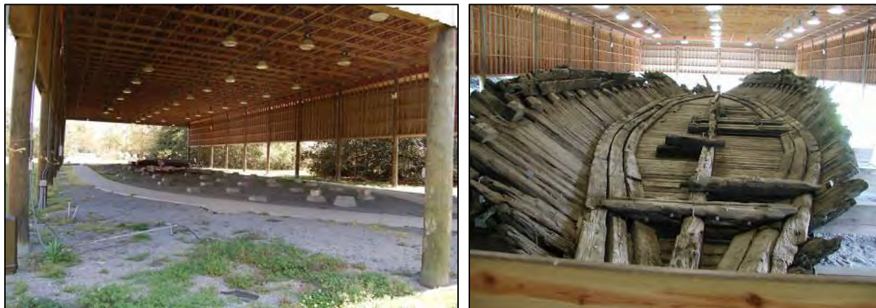
Figure 222: View looking north at interior of C.S.S. Neuse shed, at left; 2003 photograph of C.S.S. Neuse in shed, at right (courtesy of C.S.S. Neuse State Historic Site).
