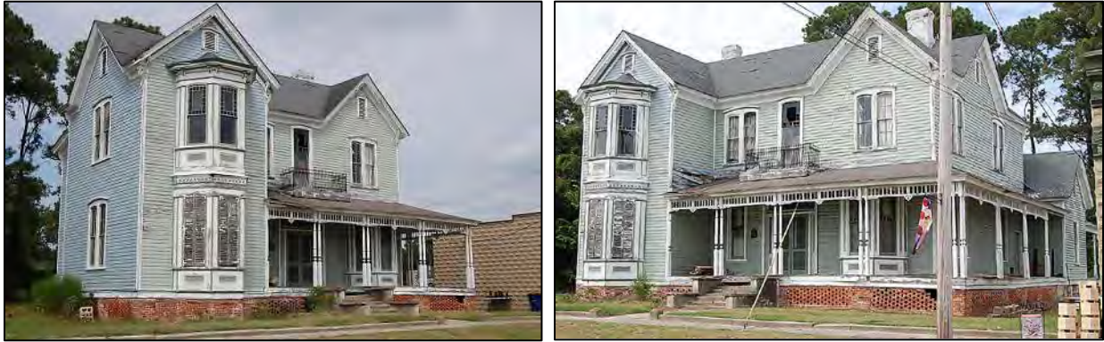
Figure 31: George B.W. Hadley House: west side and south front elevations, at left, and south front and east side elevations, at right, 2017.
