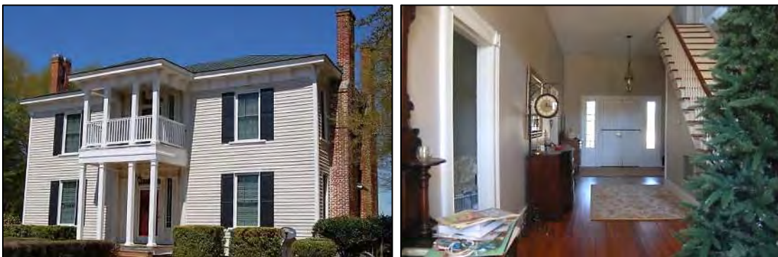
Figure 105: Dempsey Wood House: south front and east side elevation, at left, and hall and stair from front entry, at right, 2017.
