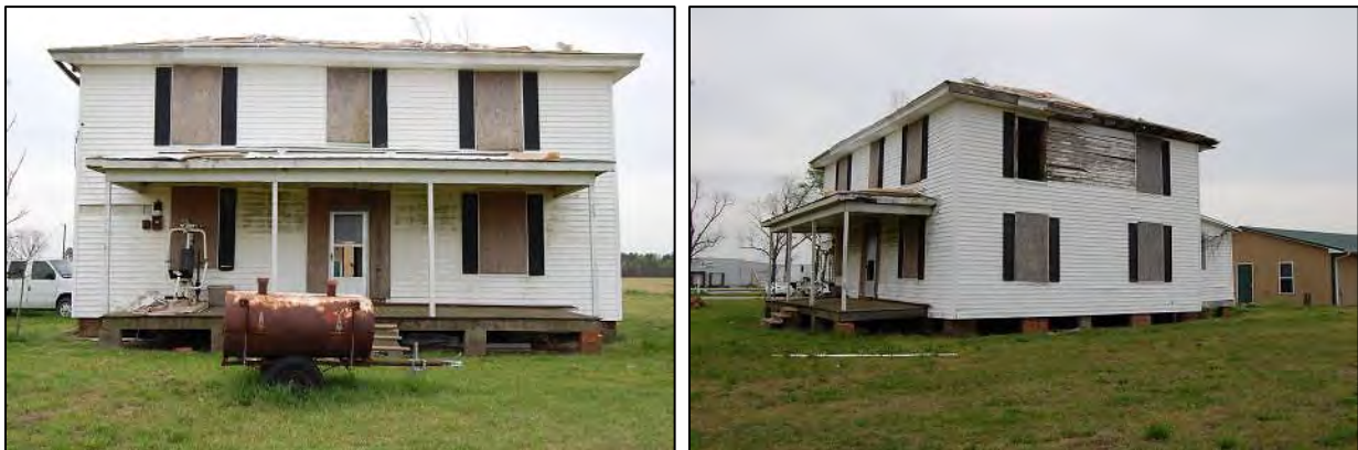
Figure 278: Robert Bond Vause House: west front elevation, at left, and west front and south side elevations, at right.
