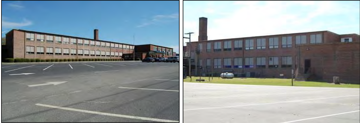
Figure 178: Woodington Middle School: at left, north front elevation of original block; at right, south rear elevation of block.
