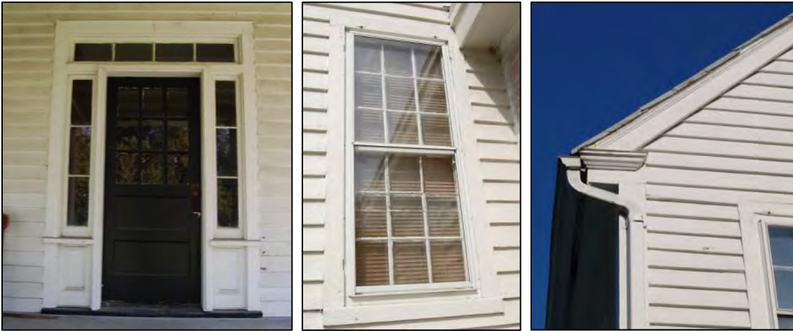
Figure 262: Left: detail of front door sidelights and transom; center: detail of original nine-over-nine light windows; right: detail of boxed cornice.
