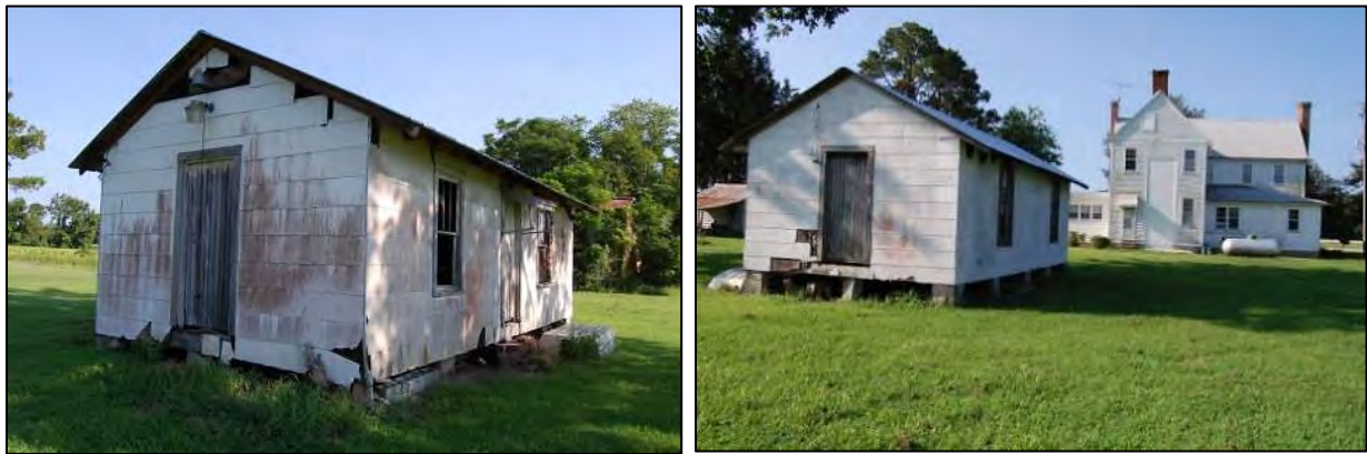
Figure 265: Left, view looking north of the storage house; right, contextual view looking south of Storage House in relation to main house.
