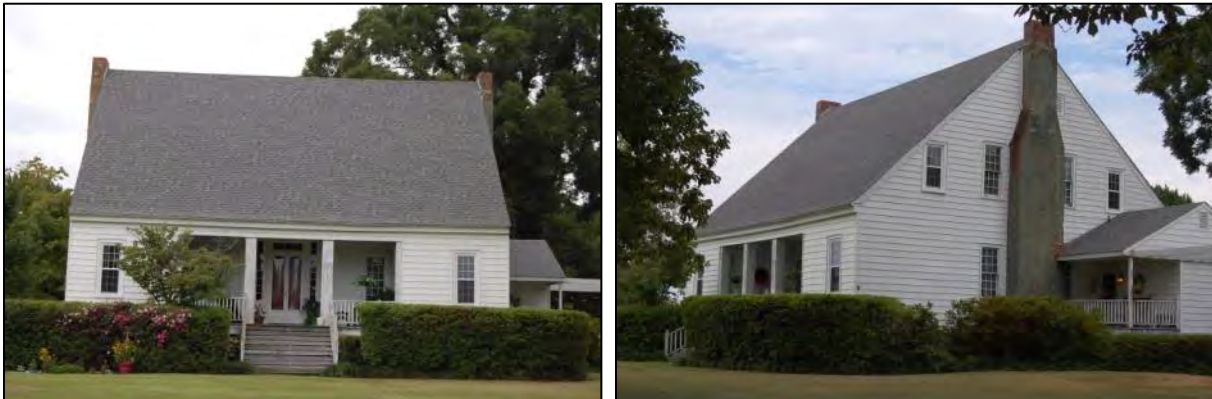
Figure 15: LaFayette: south front and east side elevations, 2017.
