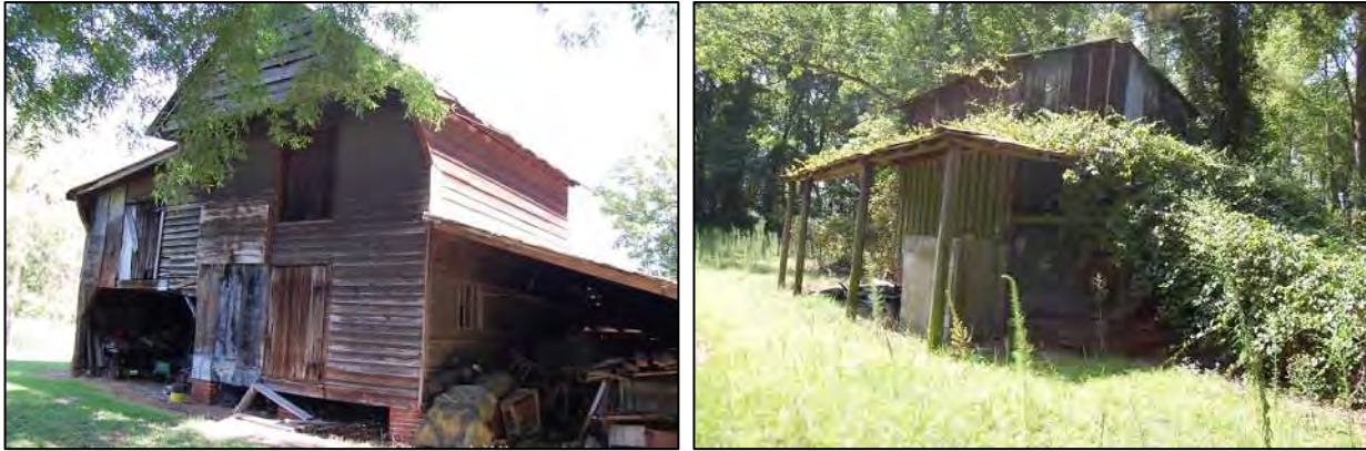
Figure 237: At left, south front and east side elevation of packhouse;; at right, view looking south of tobacco barn.
