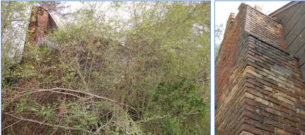
Figure 243: Moseley-Stroud House: west side elevation and chimney detail, 2017.
