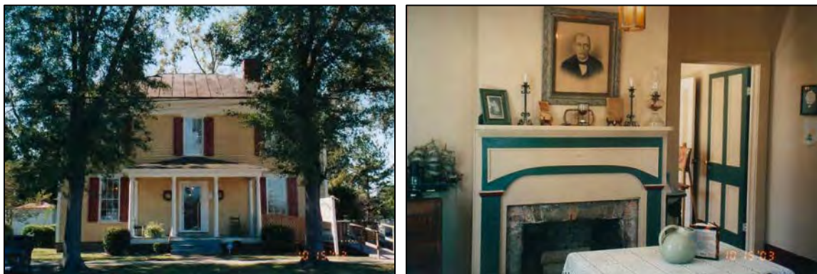
Figure 25: Archbell House/(former) Baptist Parsonage; front elevation and post-and-lintel mantel with arched panel (source: Lenoir County Historical Association, 2003).
