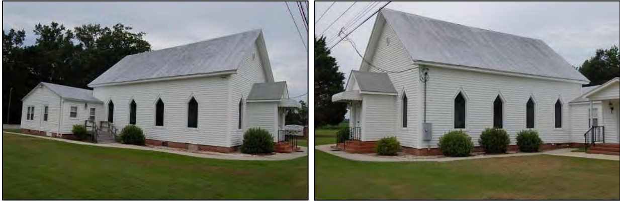
Figure 56: Bethel Christian Church: south side and east front elevations, at left, and east front and north side elevations, at right, 2017.
