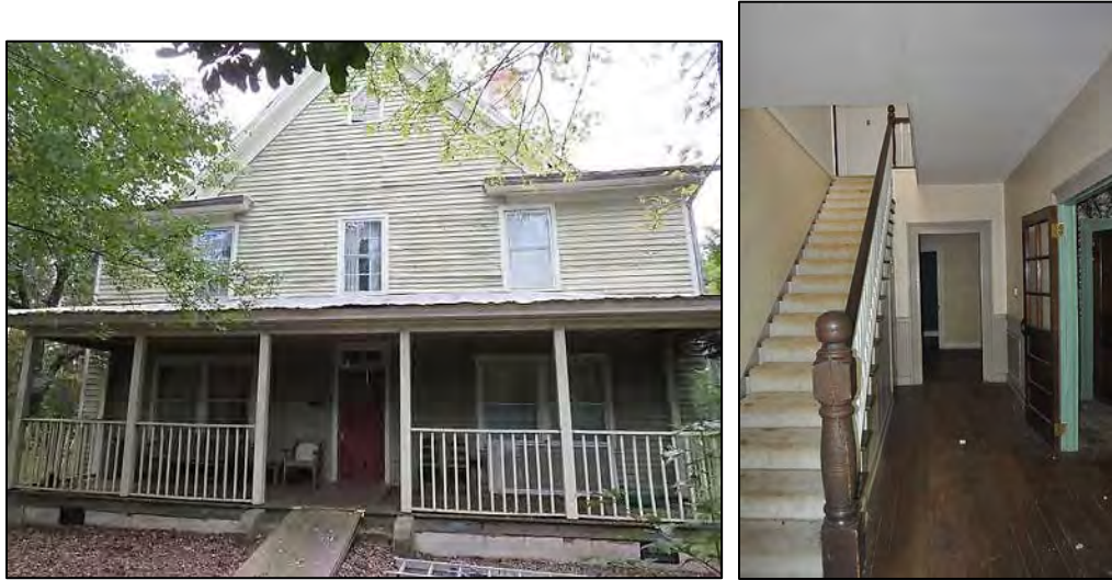
Figure 342: Leesville School Teacherage: east front elevation, at left, and interior, at right, in 2016 (source: Preservation North Carolina)
