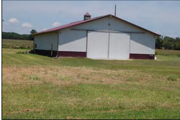
Figure 215: View of long west and gabled south elevations of modern barn.
