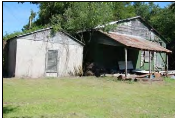
Figure 254: Frame shed adjacent to concrete block building (looking east), 2017.
