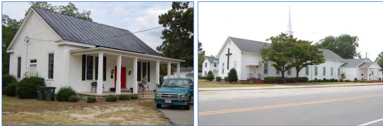
Figure 174: Bear Creek Primitive Baptist Church, east gable and long north elevations, at left; view looking west at Wheat Swamp Christian Church, at right, 2017
