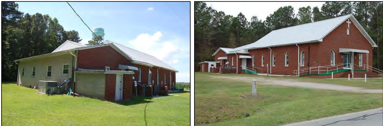
Figure 316: King's Chapel Church: at left, south rear and east side elevations; at right, east side and north front elevations
