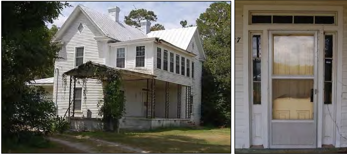
Figure 37: H. William Davis House: east side and north front elevations, and front entry with sidelights, transom, and Italianate-style paneled door, 2017.
