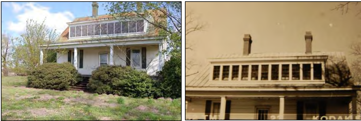
Figure 72: Warters-Parrott-Coleman House: south front elevation with boarded-over shed dormer in 2017; and shed in 1994 with at least part of roof to its rear visible through windows (Robbie Jones).
