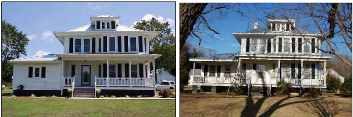
Figure 200: Simpson Waller House: at left, south front elevation in 2017 and, at right, in 2010 with chimneys, porches, and weatherboards in place.
