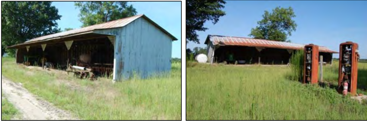
Figure 83: At left, view looking southwest at equipment shed; at right, old gas pumps a short distance to its front.
