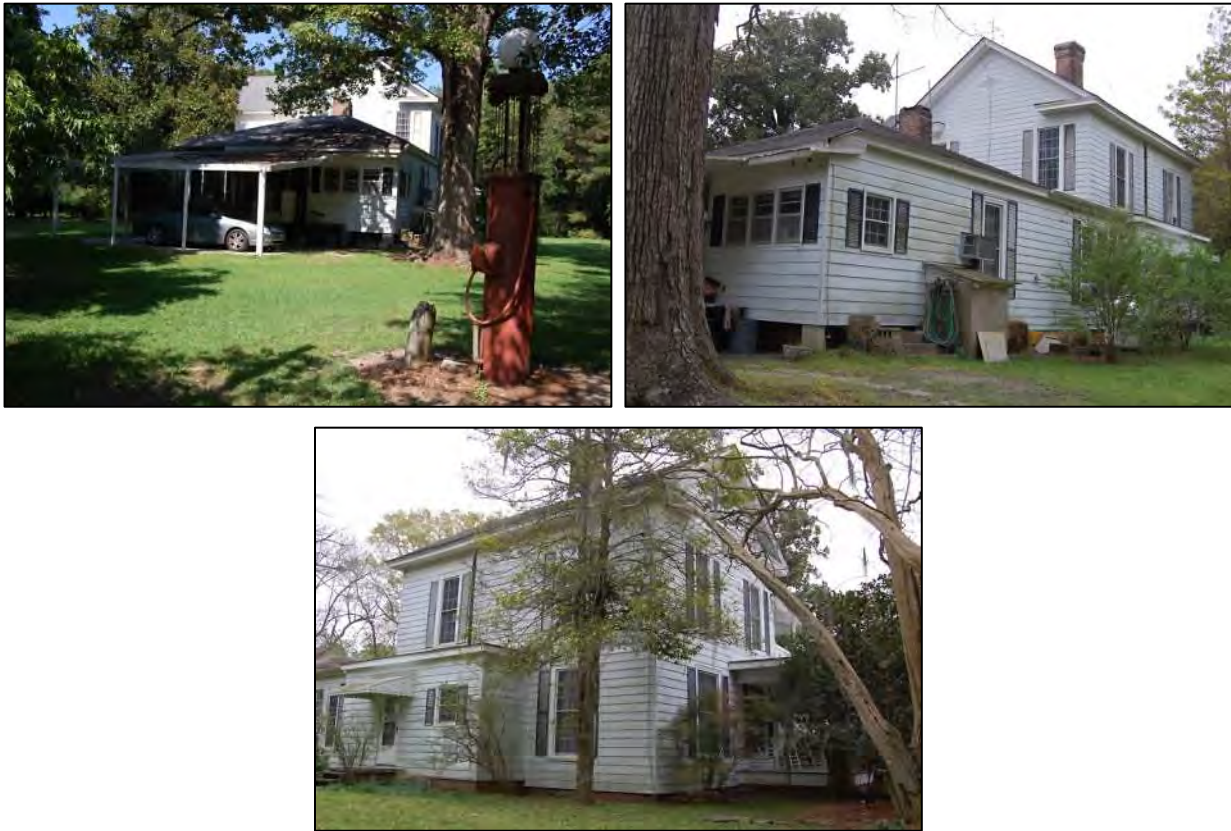
Figure 321: Elijah Loftin House: top left, east rear elevation of house; top right, east rear and north side elevations; bottom center, north side and west front elevations.
