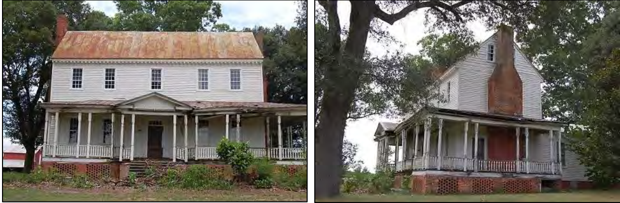
Figure 9: Herring House: south front and east side elevations, 2017.
