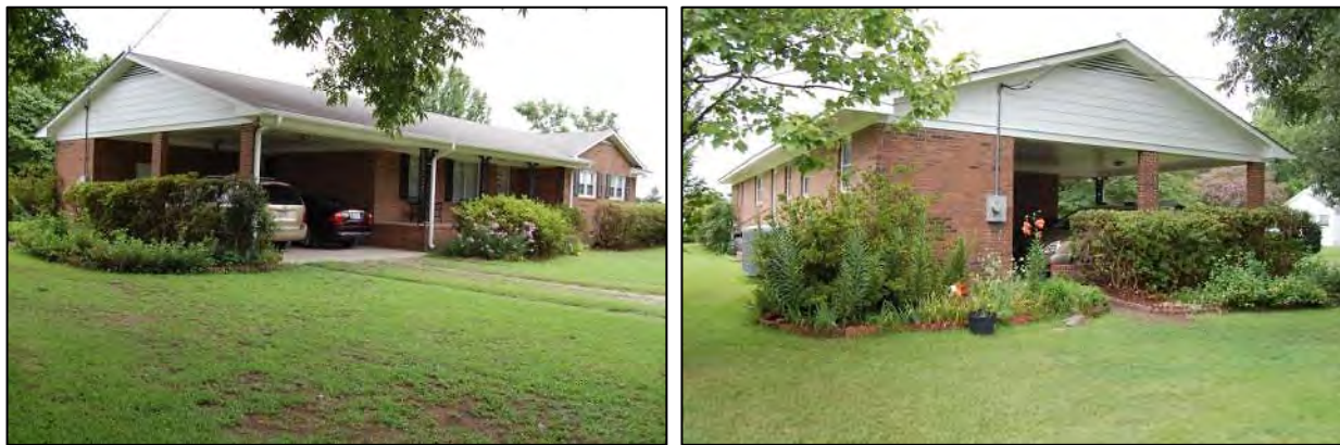
Figure 132: Billy Baker House: at left, east side and north front elevations; at right, south rear and east side elevations.
