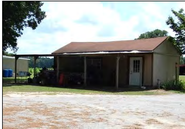
Figure 110: View of eastern elevation of shed, looking southwest.
